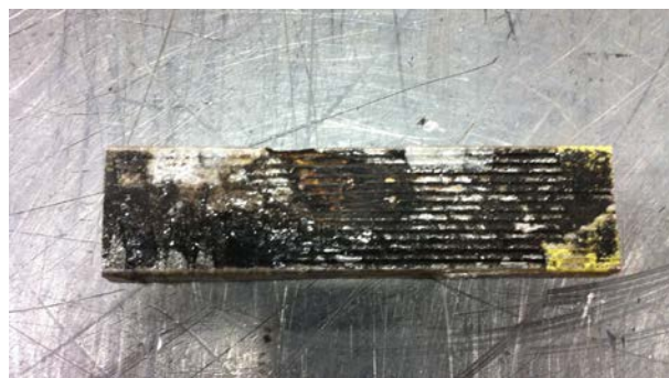
Fig. 3. Inspection of a section of failed coil after tape removal showing surface damage on conductors only indicating ground fault
