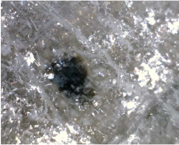
Fig. 5. Arcing point in armor tape resulting in burned mica tape.
