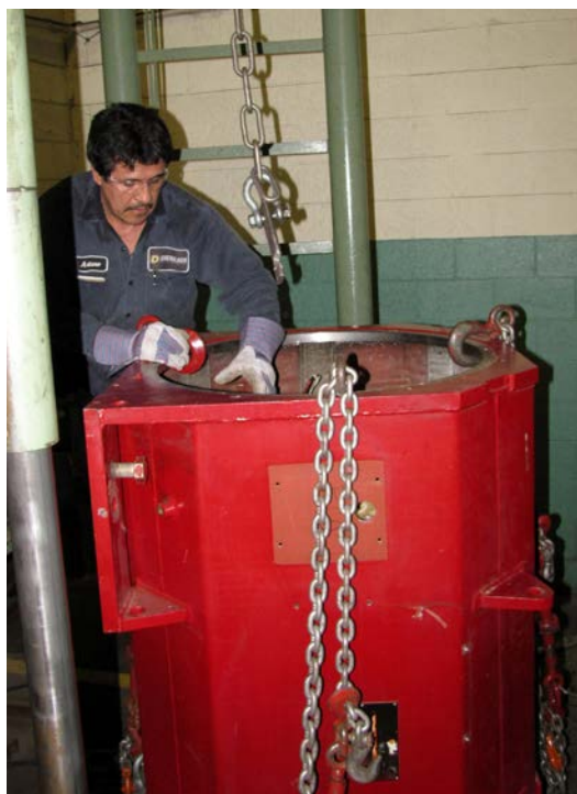
Fig. 2. Stripping Generator Vertically
